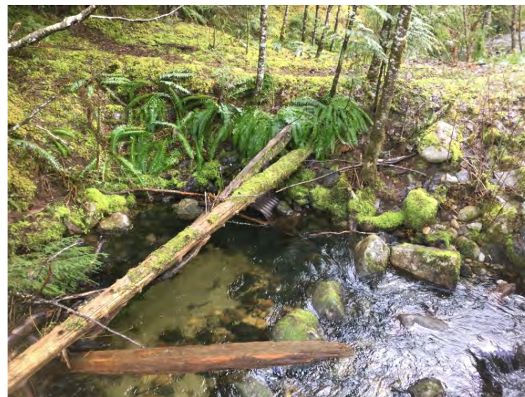
Partial flow staying on cutslope side of road flowing through CSP
