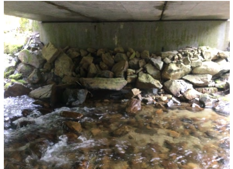
Left Bank Abutment when facing downstream
