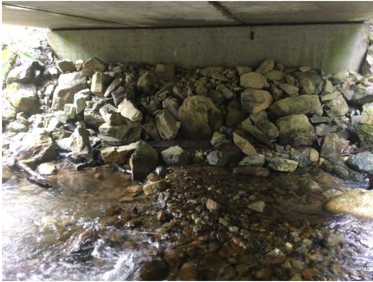
Right Bank Abutment when facing downstream
